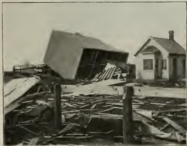
WHITE HEATH ELEVATOR AFTER THE CYCLONE.
